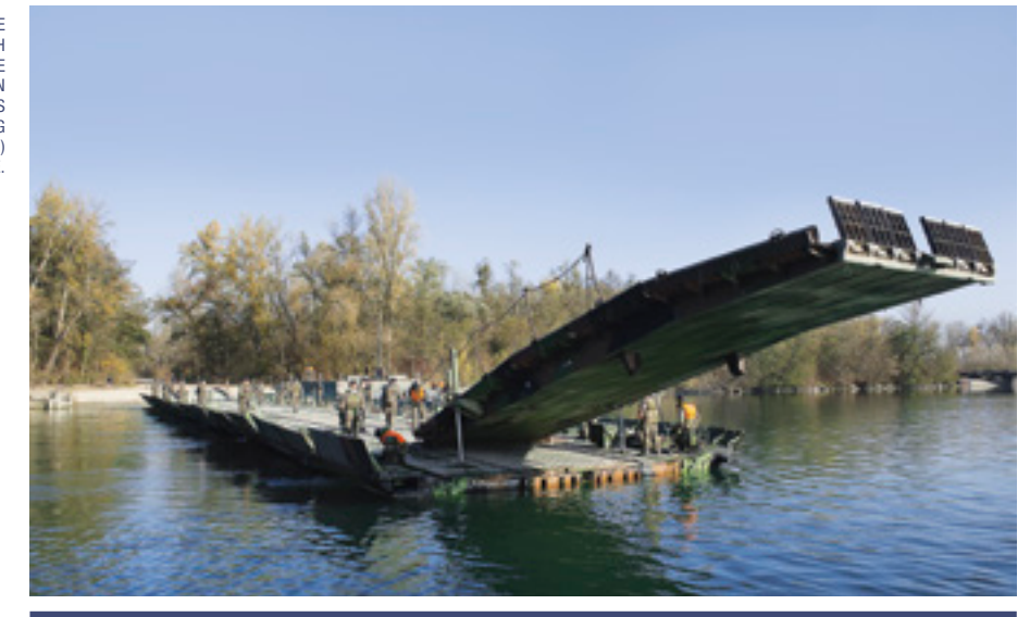
TRAINING EXERCISE BY THE FRENCH ARMY INVOLVING THE CONSTRUCTION OF 160 METERS OF MOTORIZED FLOATING BRIDGE (PFM) ON THE RHÔNE.
